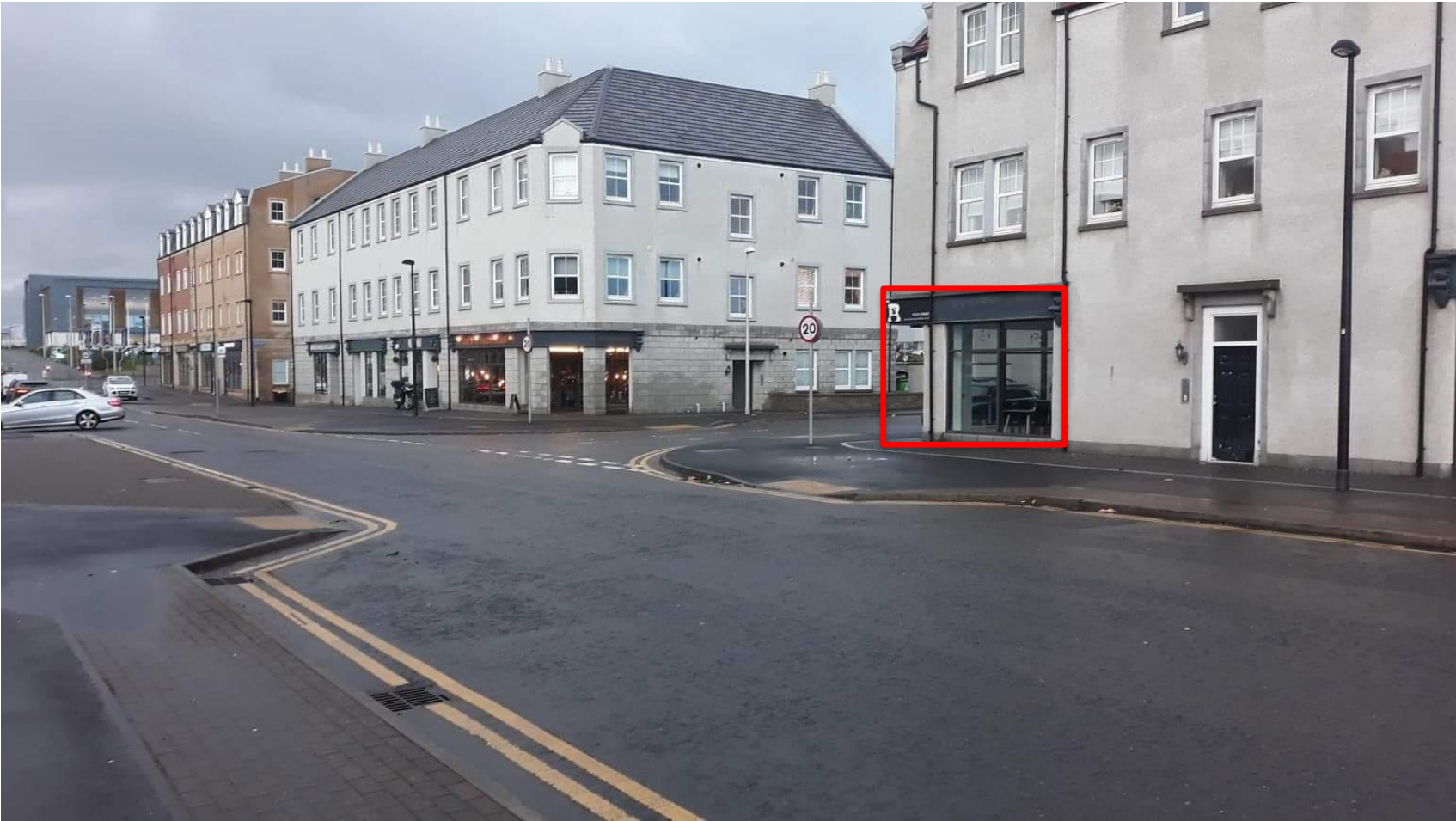
Looking West along Charleston Road North
